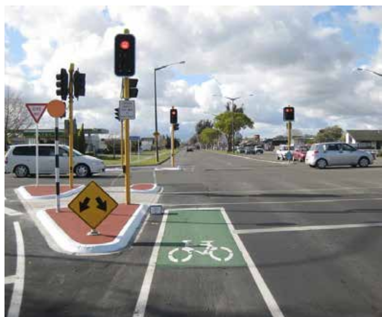
Figure 6. Example of where cycle lanes stop and force cyclists to merge with traffic on Pioneer Highway. Photo taken by student researcher.
