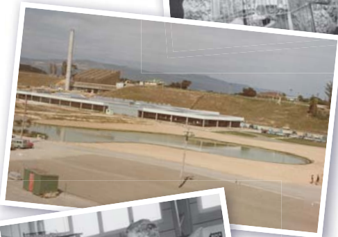
Vet clinic with lake and boiler house, 1968.
