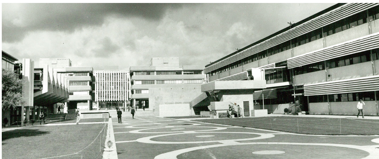
A view across the Manawatū Campus in 1969, with the Library building on the right https://tamiro.massey.ac.nz/nodes/view/932
