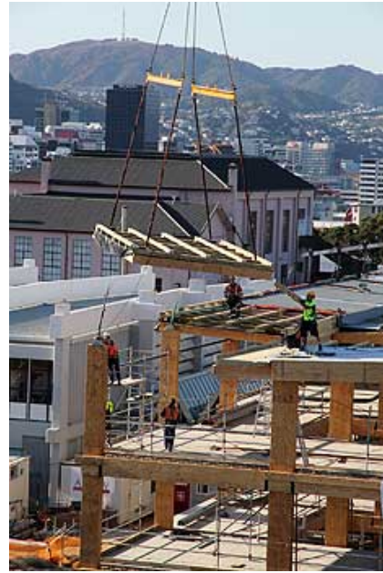
Contractors for Arrow International install a final section of the roof.
